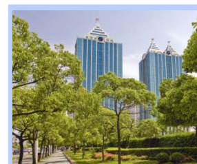
Shanghai, PRC Development Facility
